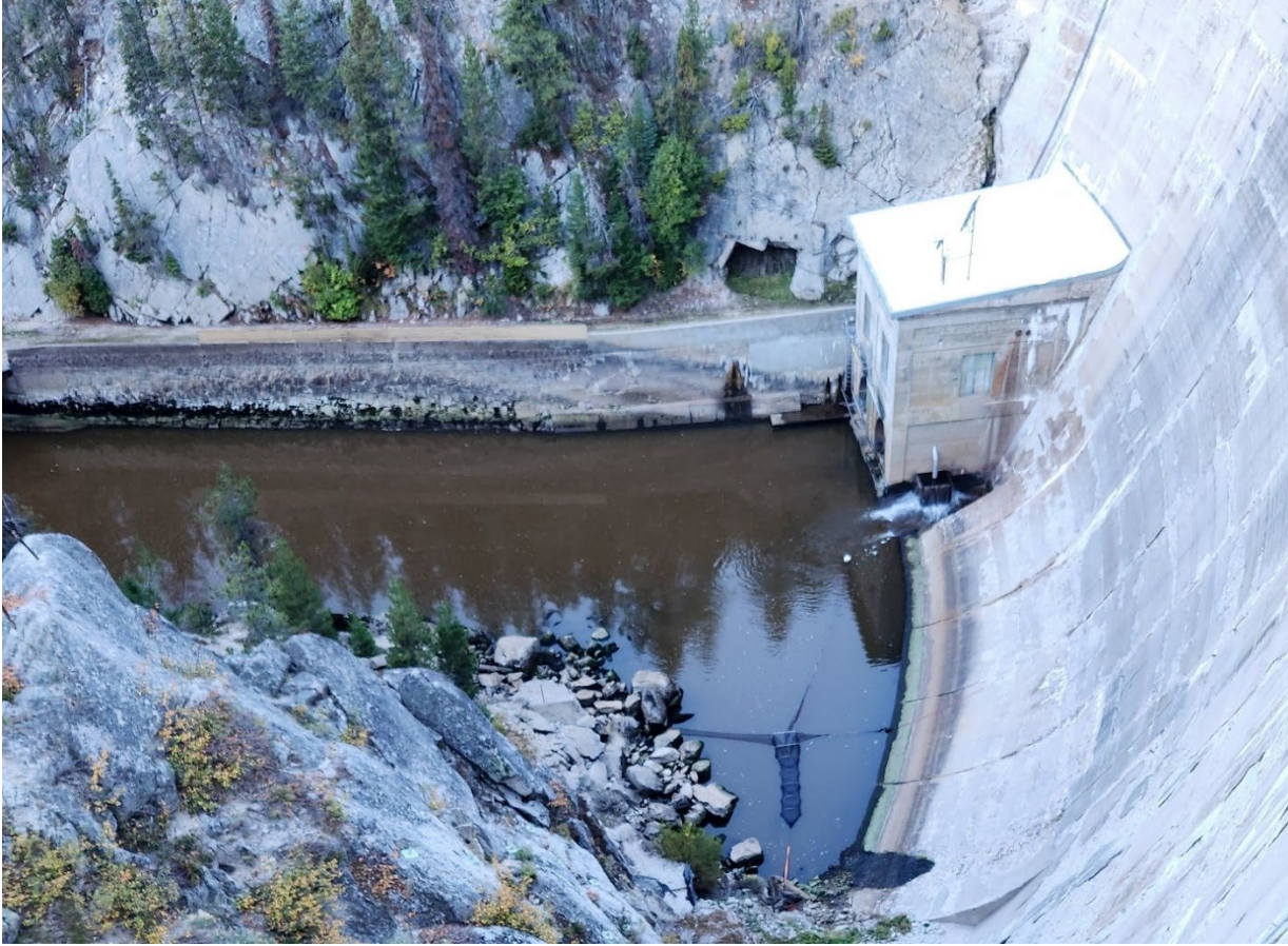
Figure 14. Fyke net location at spillway base, shoreline position. The upstream wing was attached to the face of the dam and the downstream wing was anchored to shoreline cobble. The lead line was stretched across the spillway shelf and secured to the catwalk under outlet conduits. This location worked well and should be used in the future. Note that discharge from the hydro-generator releasing approximately 2.3 cfs can be seen between the operations building and the face of the spillway.
