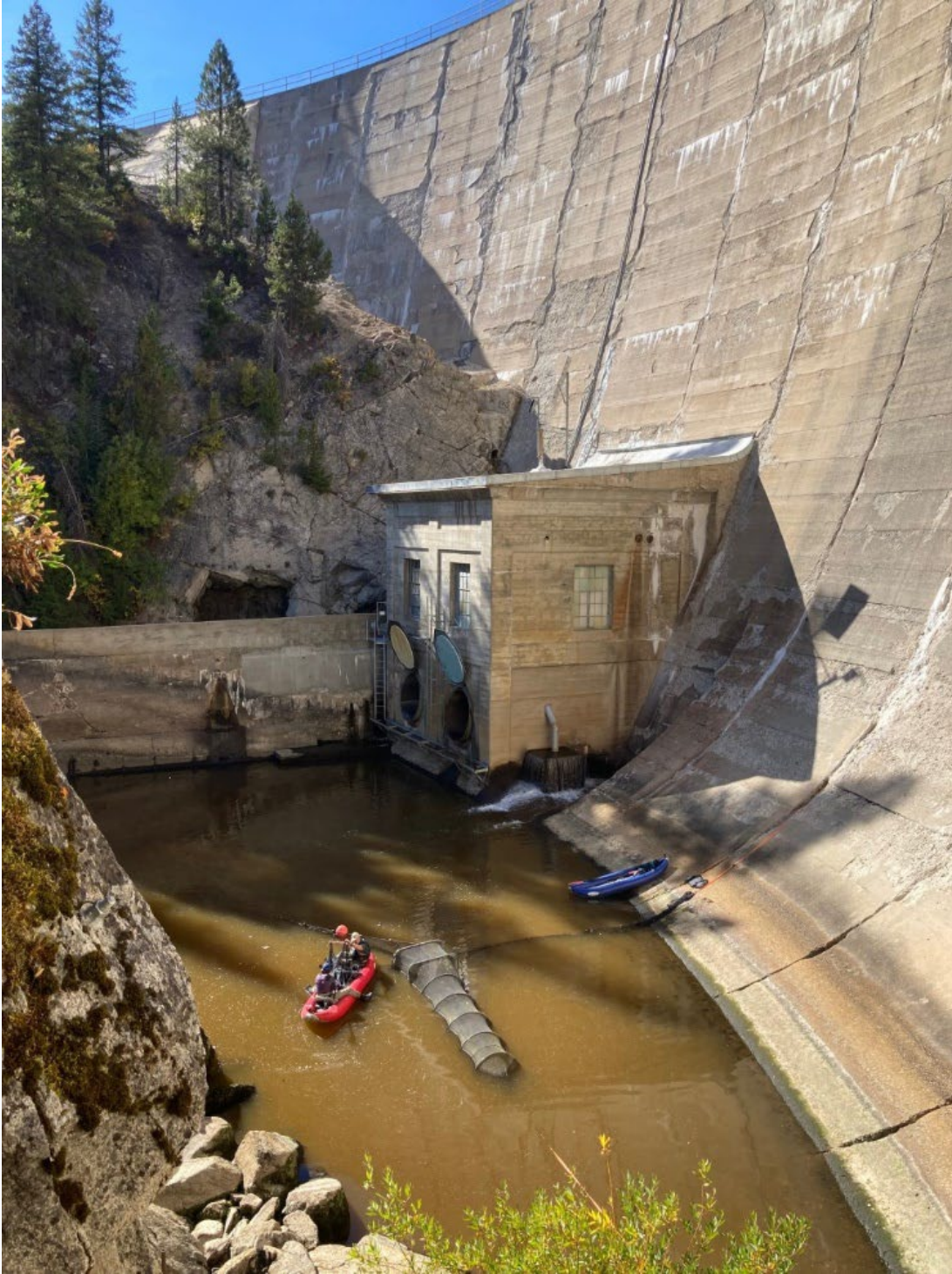
Figure 13. Fyke net location at spillway base, center position. The upstream wing was attached to the face of the dam and the downstream wing was positioned off the spillway shelf with an anchor on the lead line and a buoy with slack line attached to the float line. The lead line was stretched across the stilling basin and secured with line to the erosion wall. Note that this location was the least effective and would require adjustment if used again.
